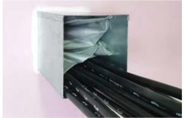
QFP QuelStop Intumescent Fire Pillows Installed in Steel Cable Trunking
